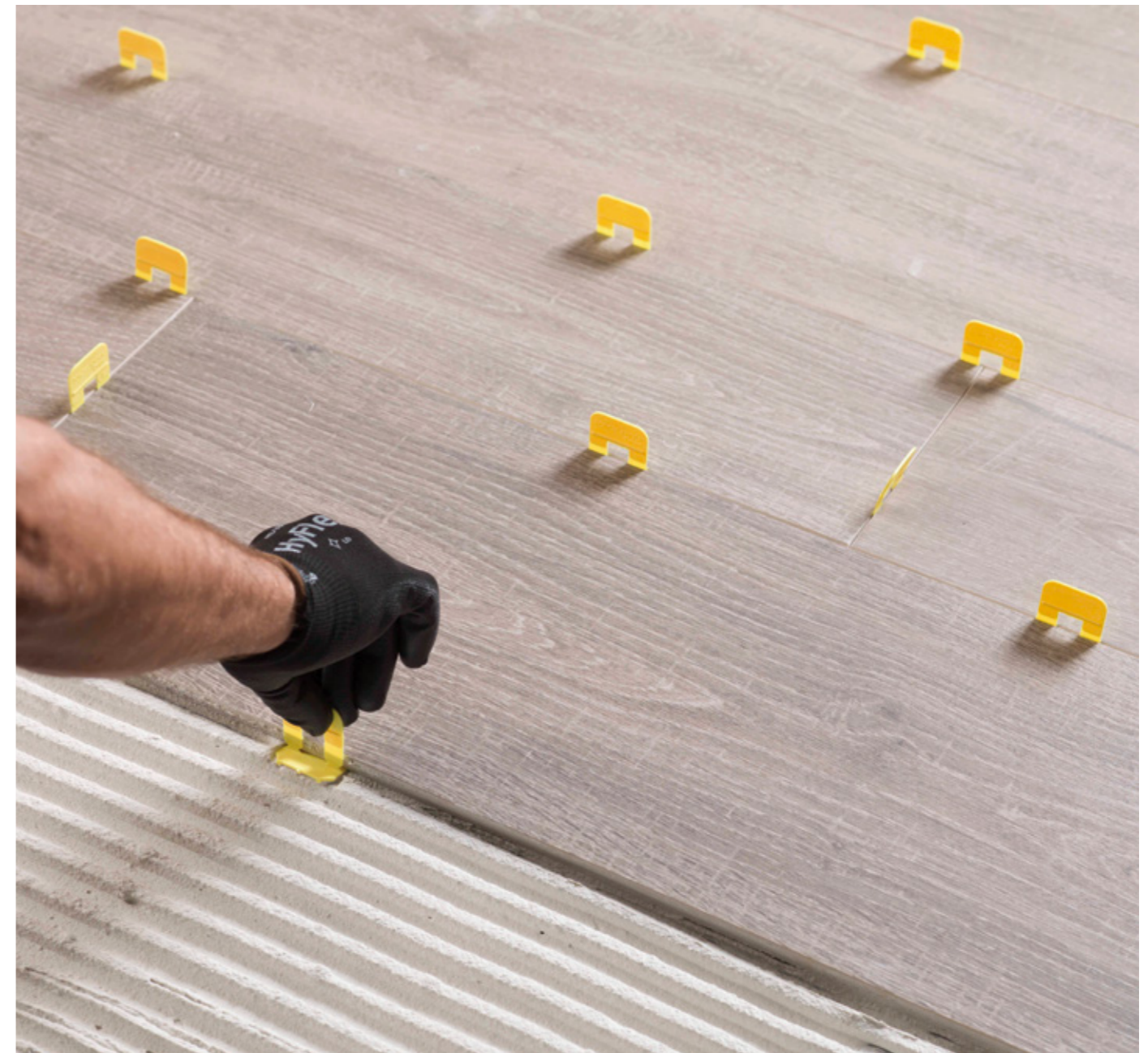
self-leveling spacers for tiles 16 to 22 mm thick
